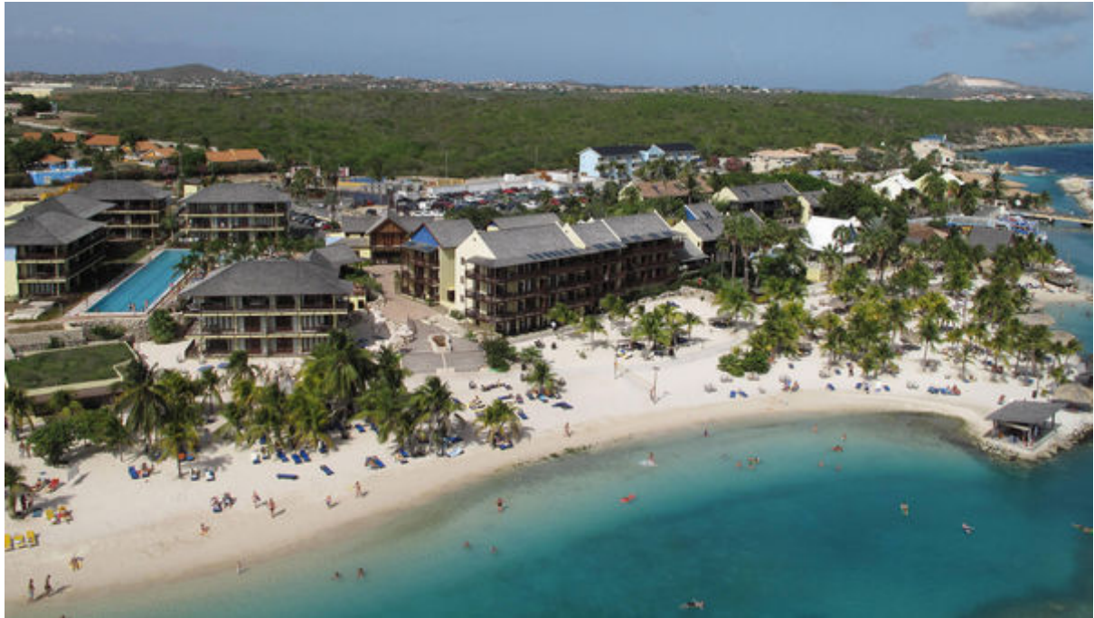
The LionsDive Beach Resort gets 70% of its daytime-use power from 600 solar panels. Photo Credit: LionsDive Beach Resort
